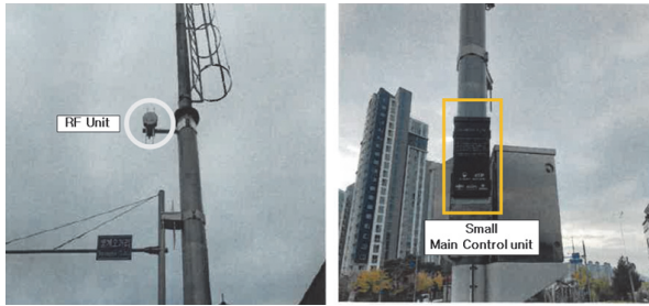
Fig. 4 RF unit and small main control unit
