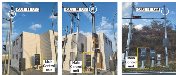
Fig. 2 RSU construction at each intersection
