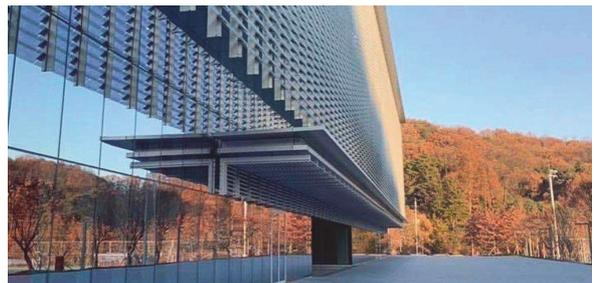
Fig. 10 Curtain wall Structure with outer reflective glass louvers, Kia Vision Square Yongin, 2021
